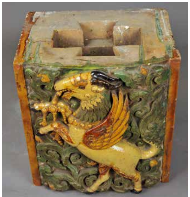
Plate 20.4 The blocks supporting the side-jamb of the arches are penetrated vertically by a stepped cavity shaped to accept a brace, strengthening the arch as a load-bearer. Nanjing Municipal Museum
