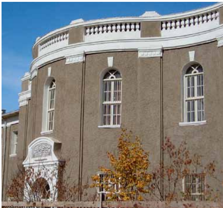
Fig. 6. Repaired exterior of the National Museum
